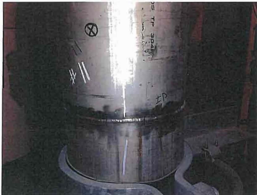
While the weld metal may not be flush with the *interior* surface, any incomplete fill will be compensated for by *external* reinforcement making the weld at least as thick as the parent metal thickness.
